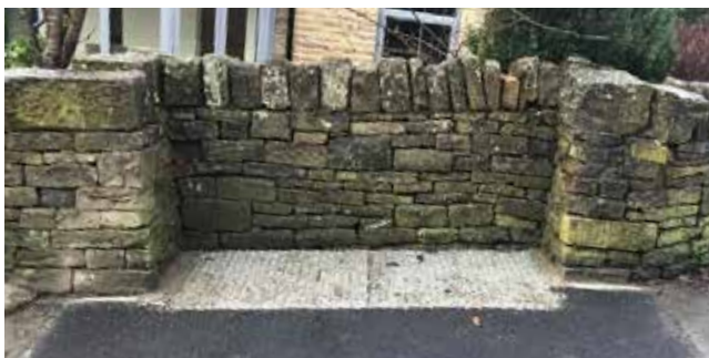
Bespoke cover installation
